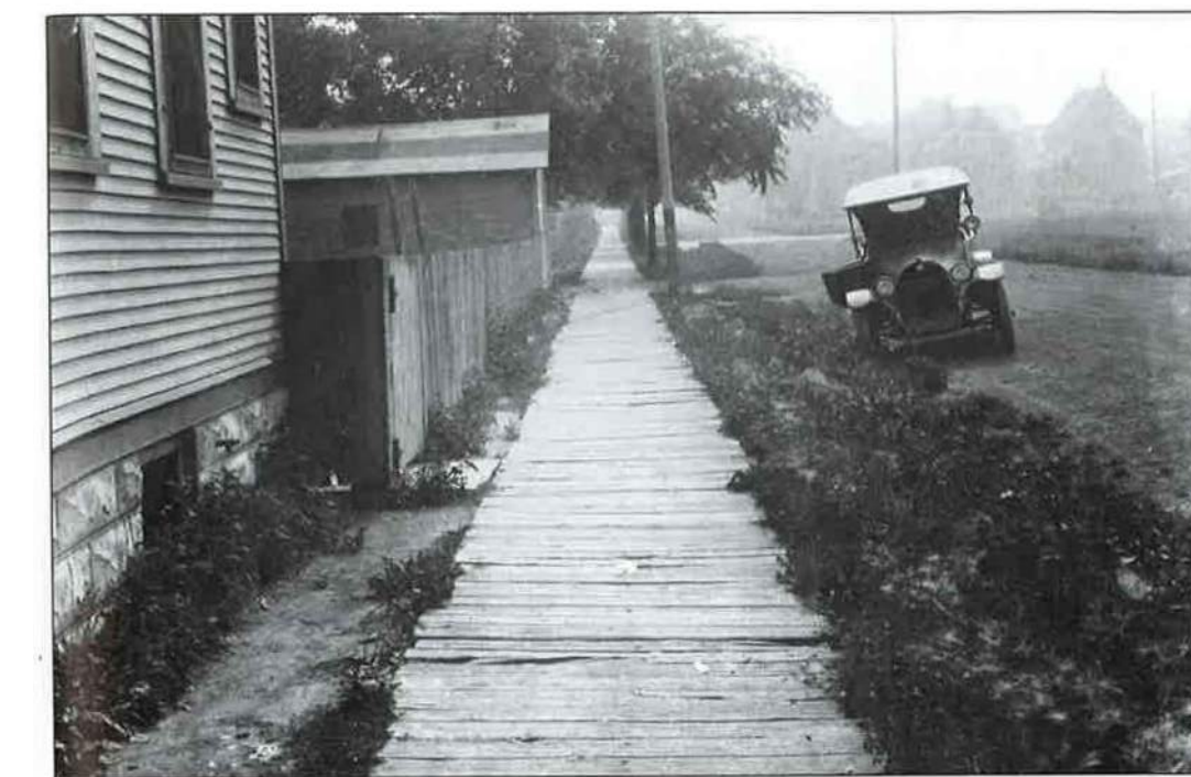
WOODEN SIDEWALKS, 1919. The older sections of West Allis were lined with wooden sidewalks. This walkway in William Shenners subdivision, east of South Sixtieth Street and north of National Avenue, shows the unevenness and problems of a wood sidewalk. In the 1920s, the city gave homeowners a tax incentive to repair the sidewalks. Maintenance was an ongoing issue and concrete sidewalks replaced many of them in the 1930s.
